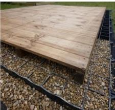
If your **ProBASE** is larger than your building you can create a French Drain by filling the excess **ProBASE** with decorative pea gravel. This helps to prevent rain water and soil splashing back onto your timbers
