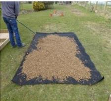
If you are finding it hard to create a level sub-base, pour 10mm round pea gravel over the membrane and rake level
