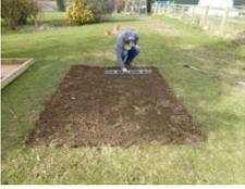
Prepare a firm, level area slightly larger than the size of your **ProBASE**. **ProBASE** can be laid directly onto grass, gravel or compacted soil.
